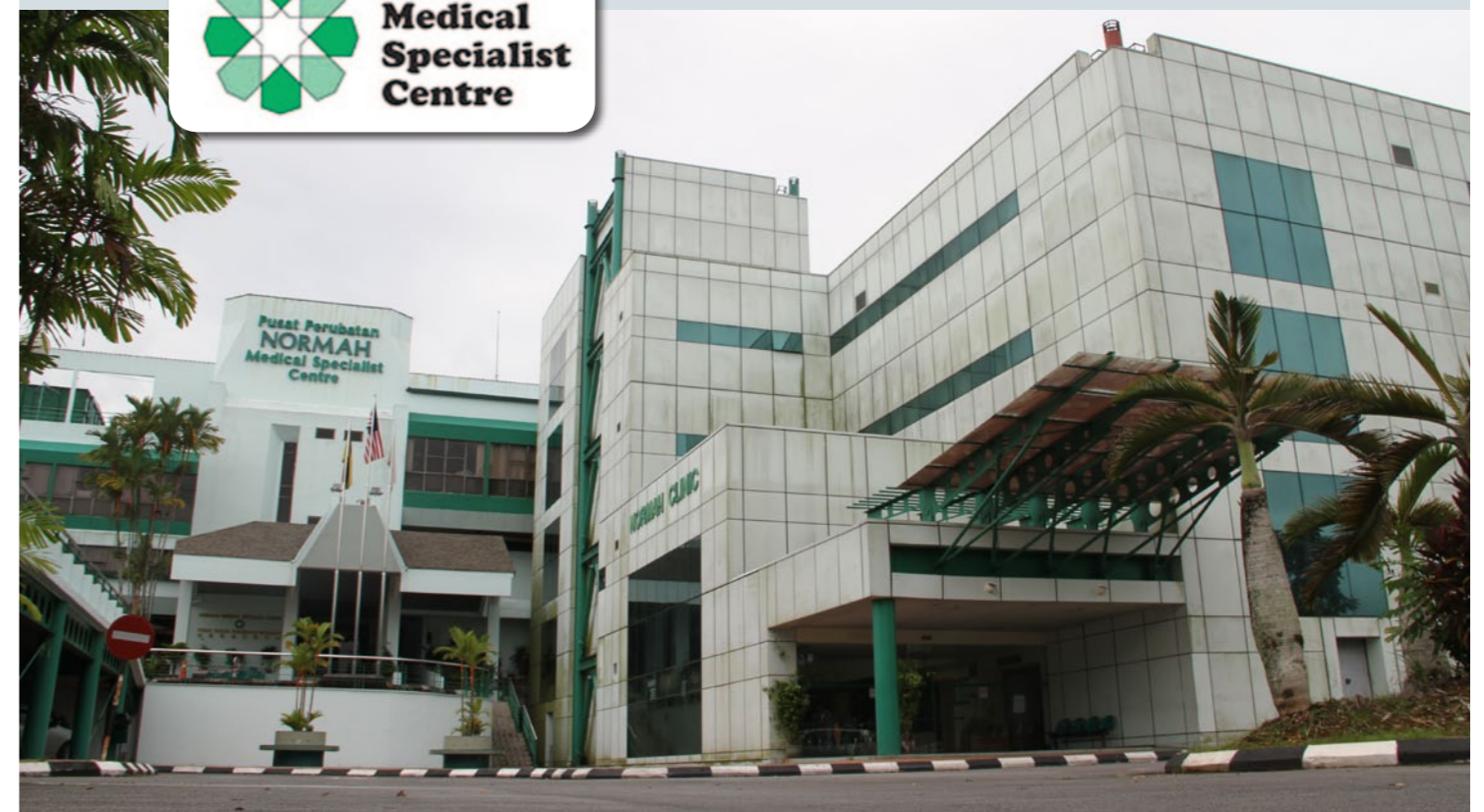
Building entrance of Normah Medical Specialist Centre (NMSC)
